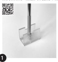
Fix Lens clips with suitable screws (min. 3 clips per metre/40").
