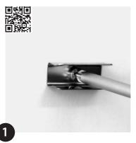
Fix clips with suitable screws (min. 3 clips per metre/40").
